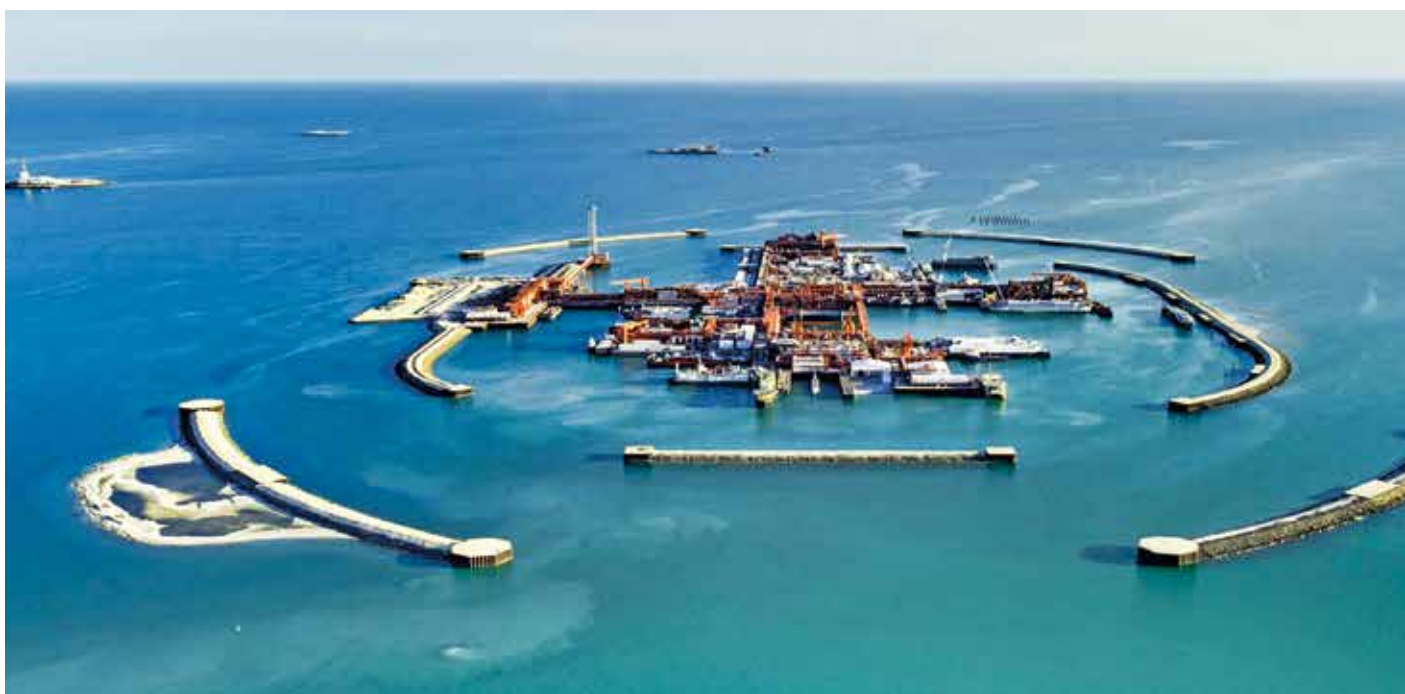
D-island, one of the artificial islands at the field of Kashagan, Kazakhstan
