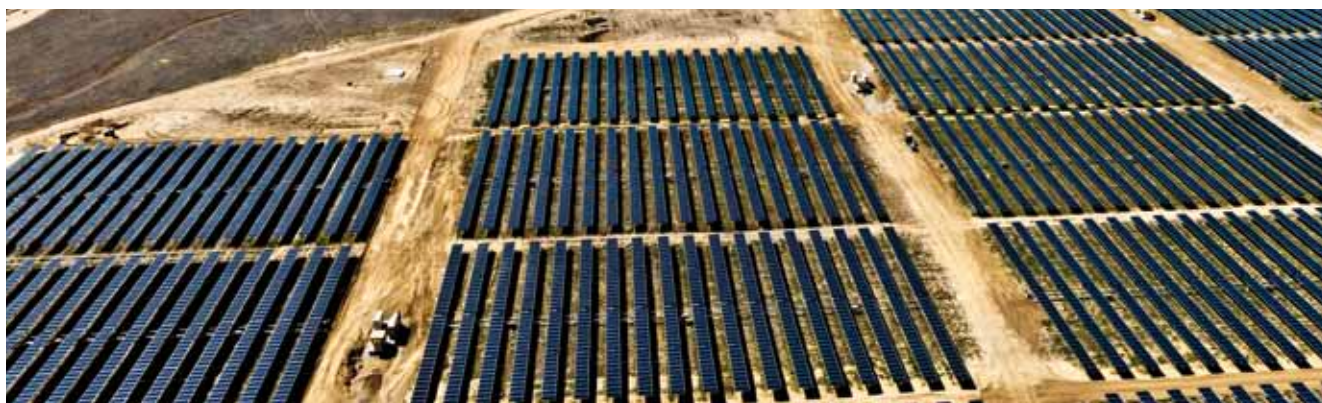
Solar panels developed by SunPower Corp., California Valley Solar Ranch, USA.
