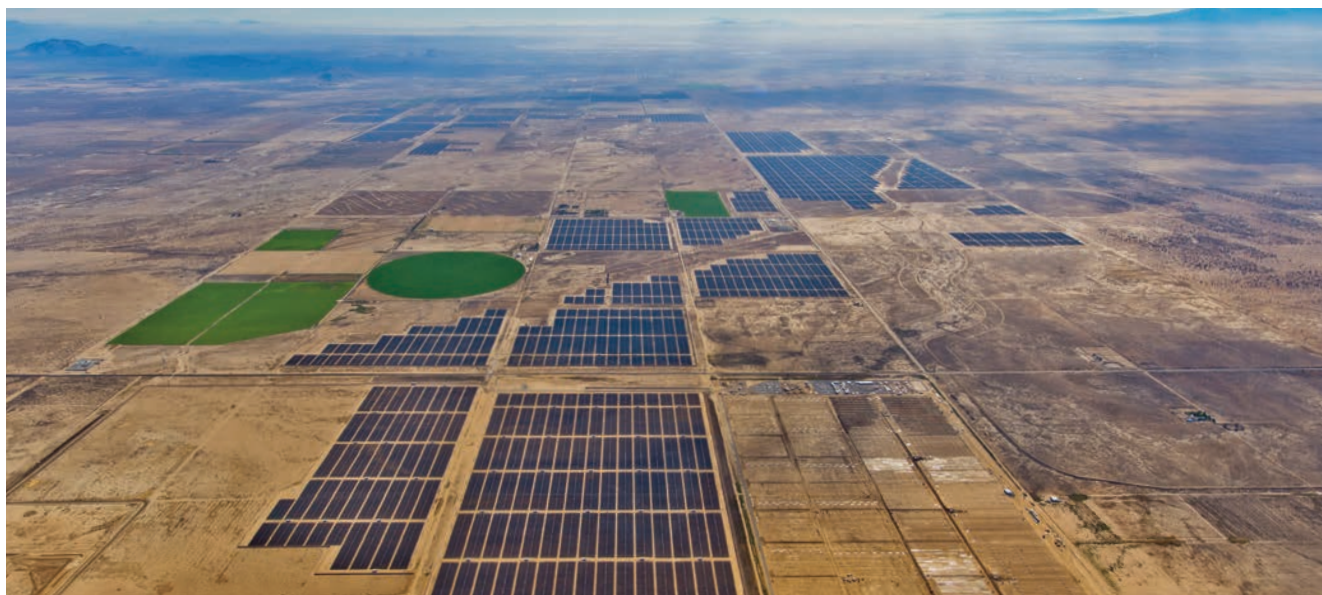
Centrale photovoltaïque SunPower Solar Star, Californie.
