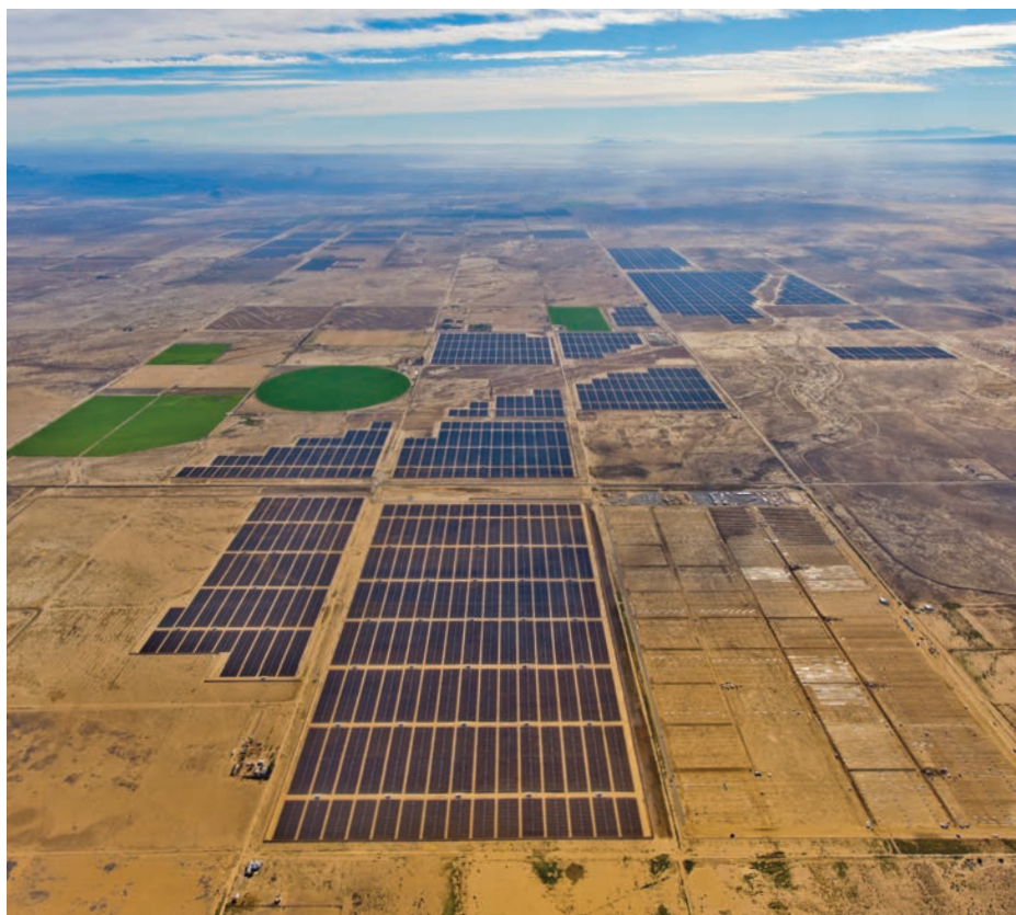
Centrale photovoltaïque SunPower Solar Star, Californie.
